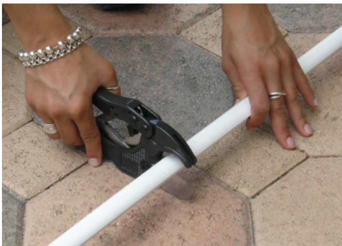
3. Cut Track Cover with a PVC cutter
